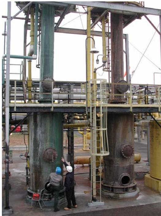
Photo 1. Akzo Nobel chemical tank T-40 captured in an FRP shell, diameter about five feet, with engineer pointing to the part to be inspected. The internal blisters are located just below the catwalk, where the shell necks down into a narrow cylinder. A man-lift was required to reach the zone to be tested.
